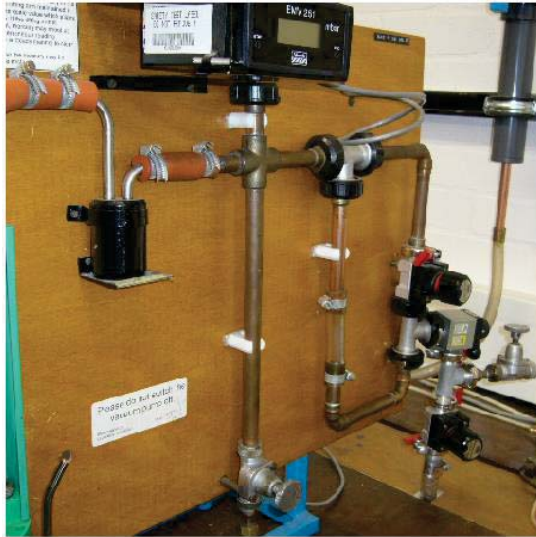
Fig 3. Pipe system as used during the experiment.
